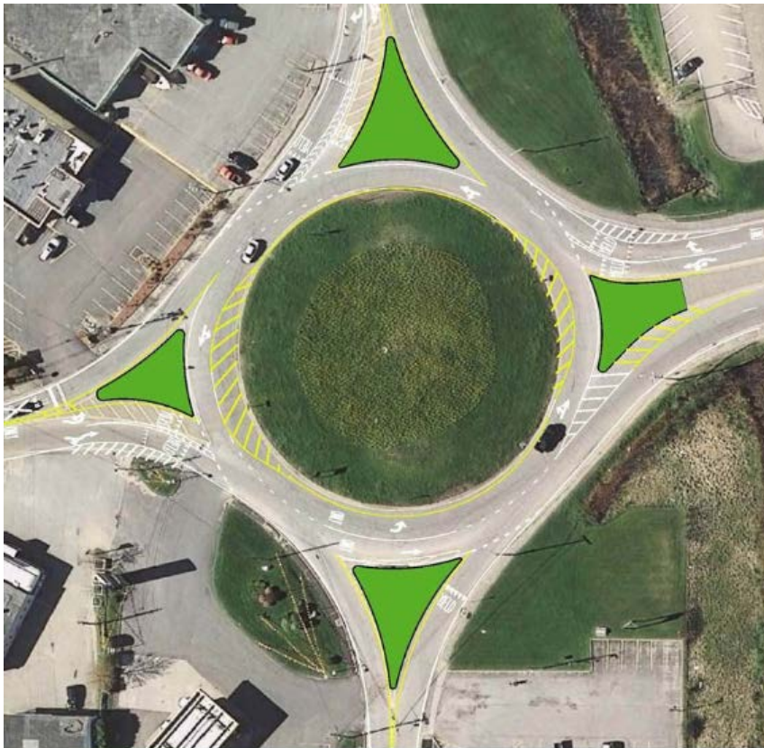
Source: Pell Bridge Design Study Report, Rhode Island Department of Transportation, 2013.
